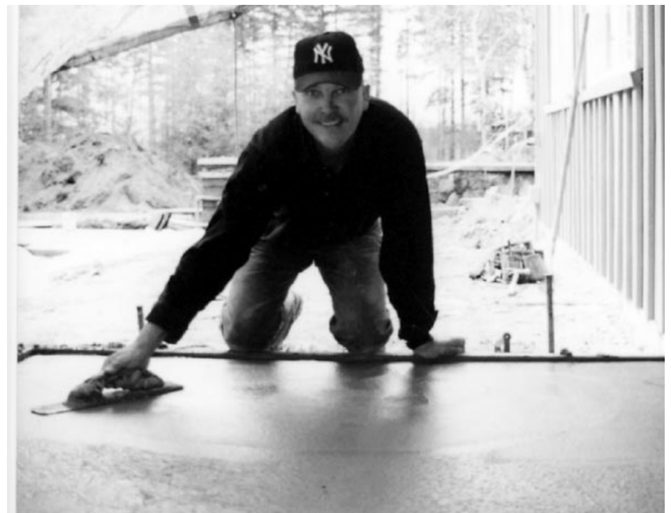
Crew Supervisor Randy Goertz finishing cement work at the new wing entrance Photo: Tanya Storr
