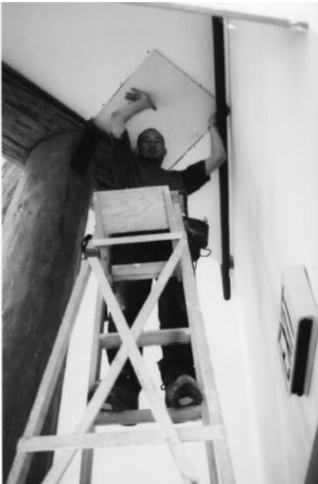
Dave Hodges installing an access hatch photo: Tanya Storr
