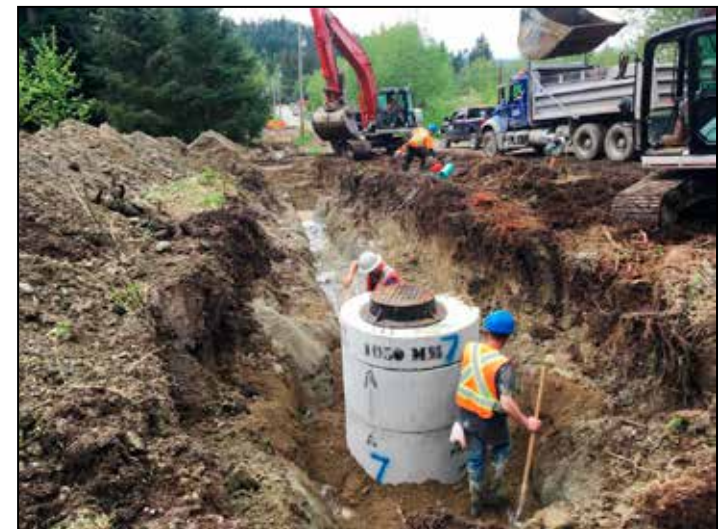
Installation of manhole and sewer line on Anderson Road.
